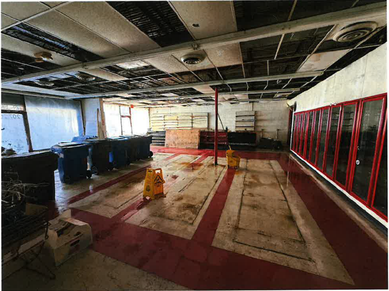
Photo 3: 205 S Wilmington Raleigh, NC (03/19/2026) Interior Facing North toward 201 S. Wilmington St.
