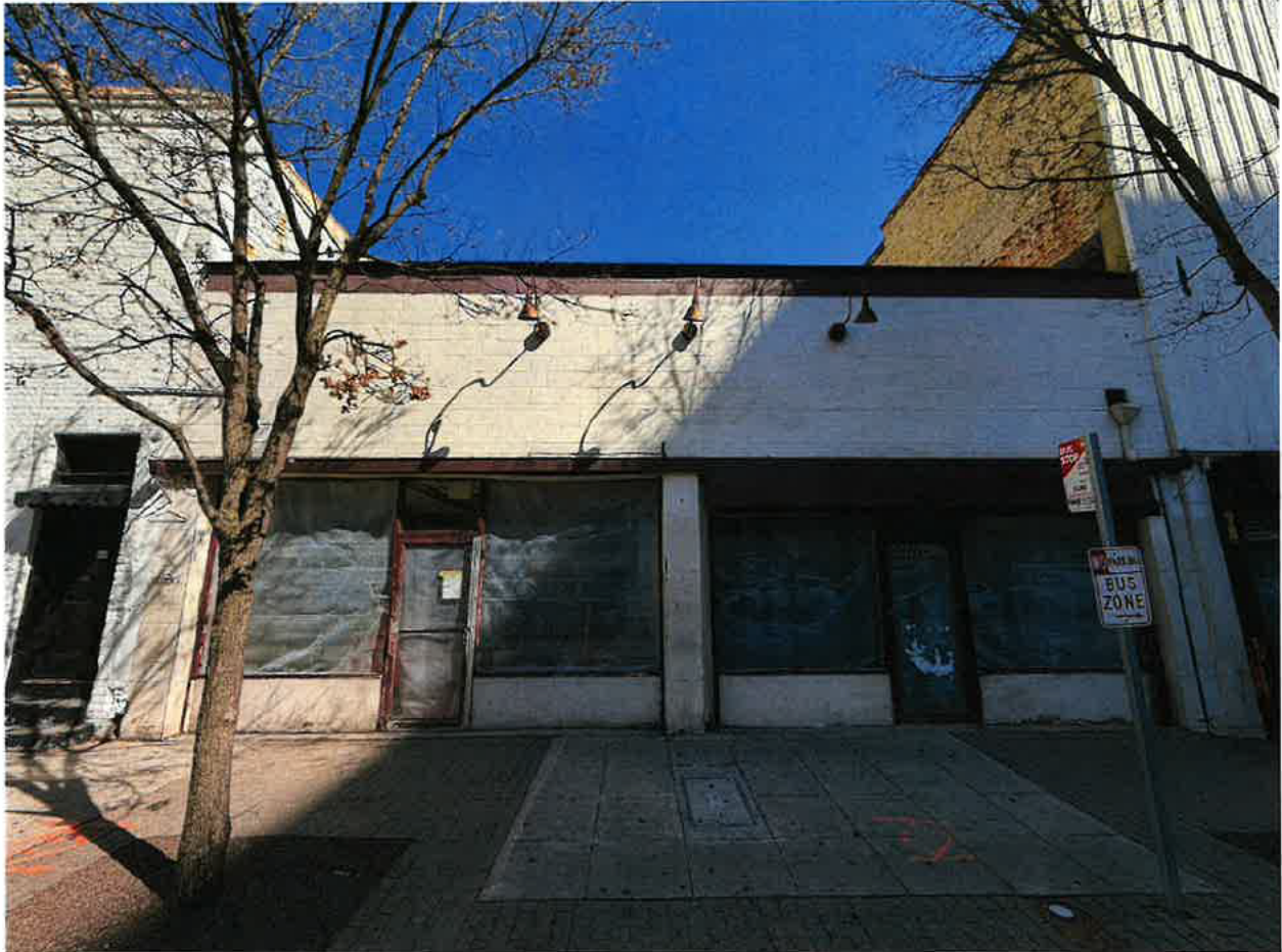
Photo 1: 205 S. Wilmington St. Raleigh, NC (03/09/206) Front Façade
