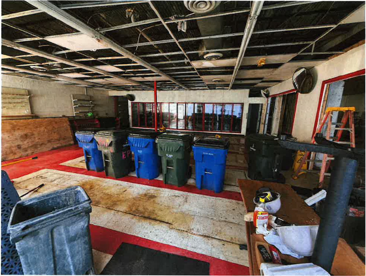
Photo 2: 205 S. Wilmington Raleigh, NC (03/19/2026): Interior Facing East
