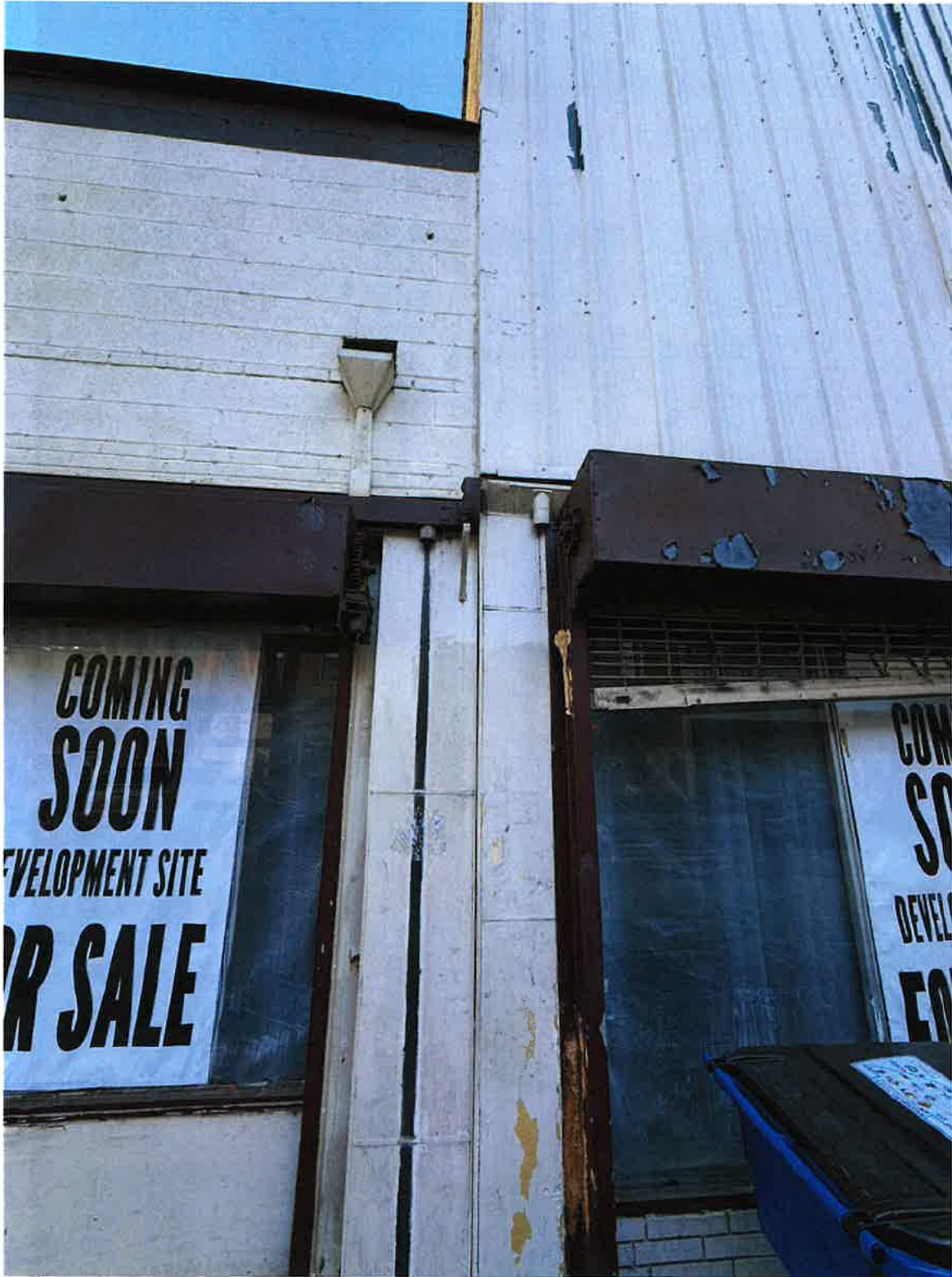
Photo 8: 205 S. Wilmington St Raleigh, NC (03/19/2026) 209 S. Wilmington structure and cladding appear to be independent of 205.
