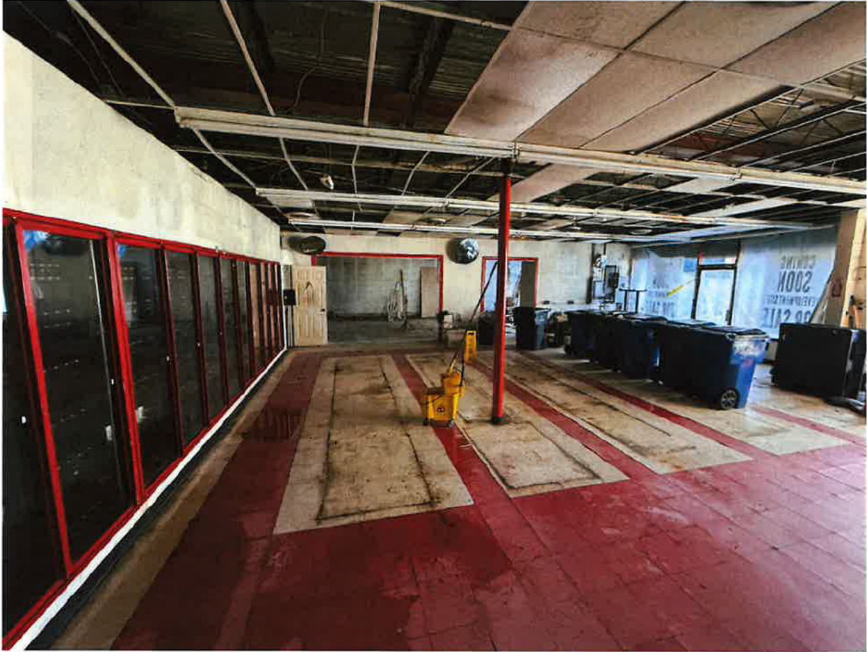
Photo 6: 205 S. Wilmington Raleigh, NC (03/19/2026) : Interior Facing South (looking into 209 S Wilmington)
