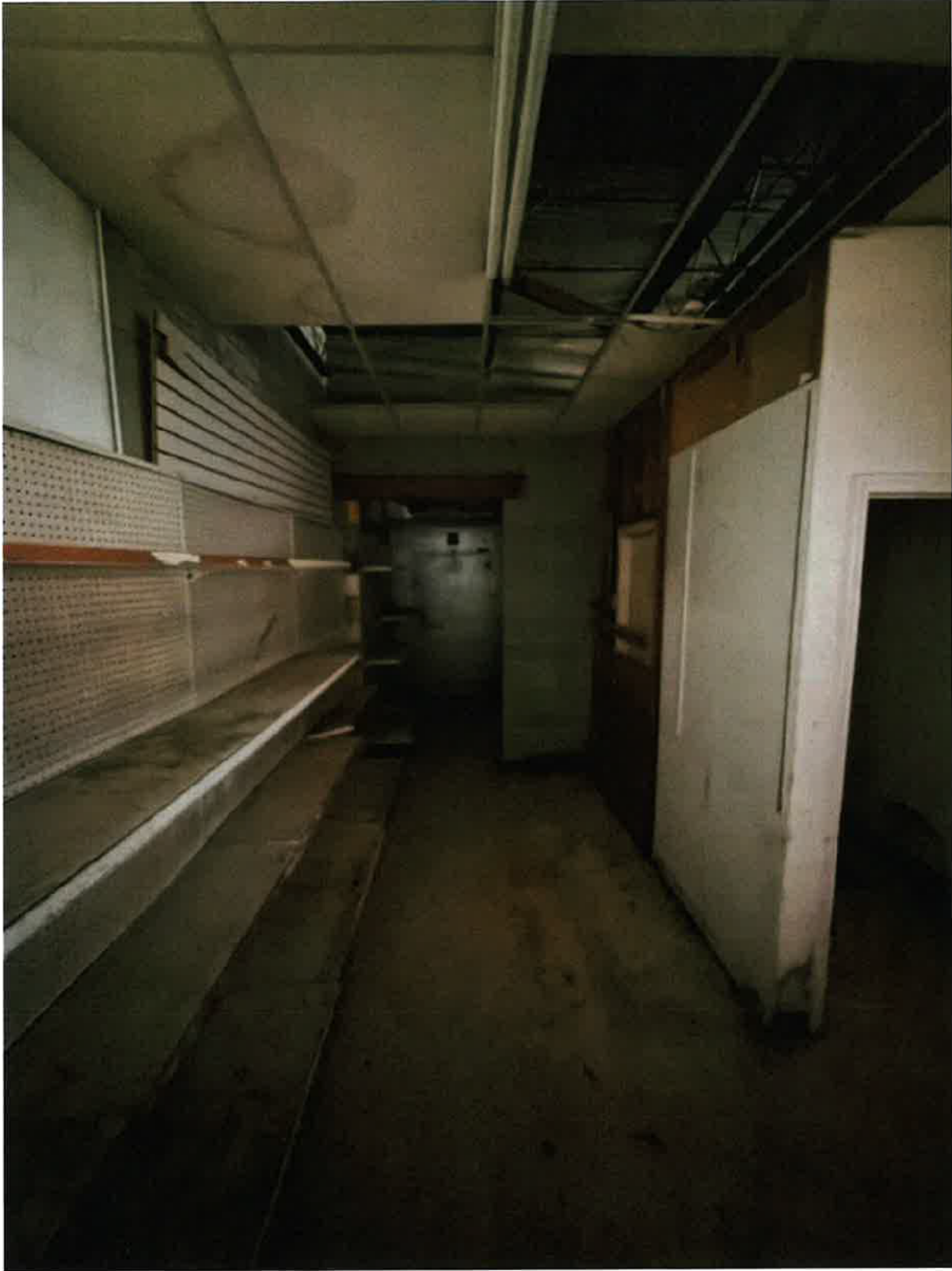
Photo 5: 205 S. Wilmington Raleigh, NC (03/19/2026) Interior, back of coolers, facing South toward rear alley of 209. No access.
