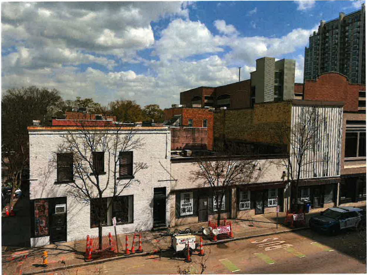
Photo 3: 209 S. Wilmington St. Raleigh, NC (03/19/2026) View from 20 E Hargett St Rooftop
