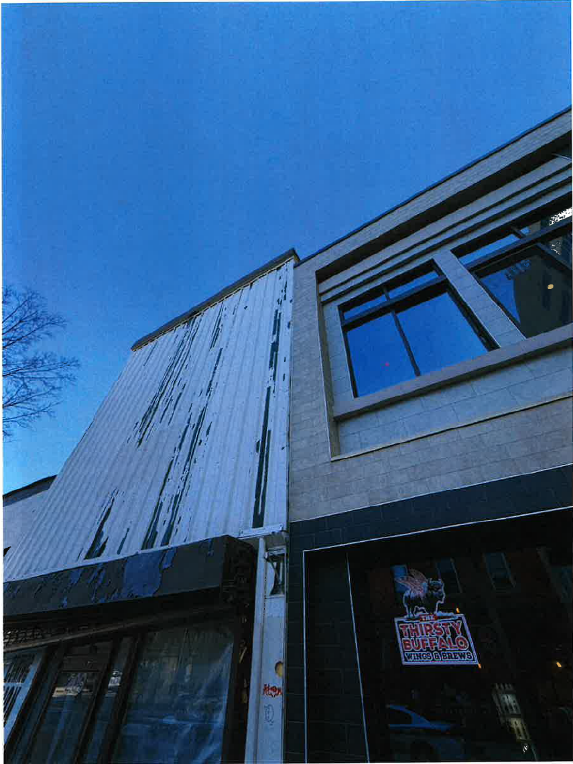
Photo 21: 209 S. Wilmington St Raleigh, NC (03/19/2026) 209 S. Wilmington St. and 211 S. Wilmington facades appear to be structural independent.
