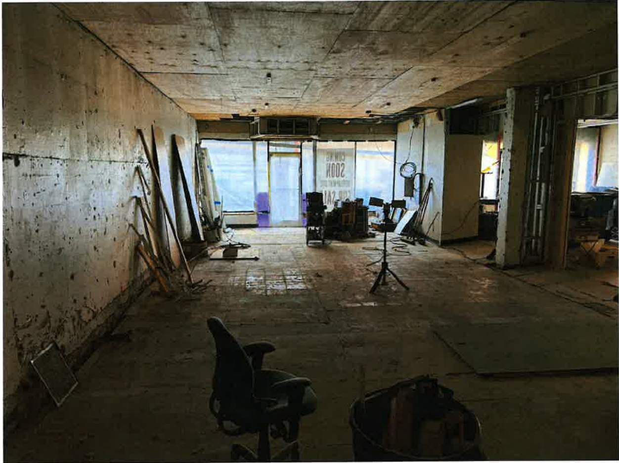
Photo 5: 209 S Wilmington Raleigh, NC (03/19/2026) 1 st floor, Interior Facing West. In addition to the original storefront, much of the first-floor framing has been replaced and none of the original flooring remains.
