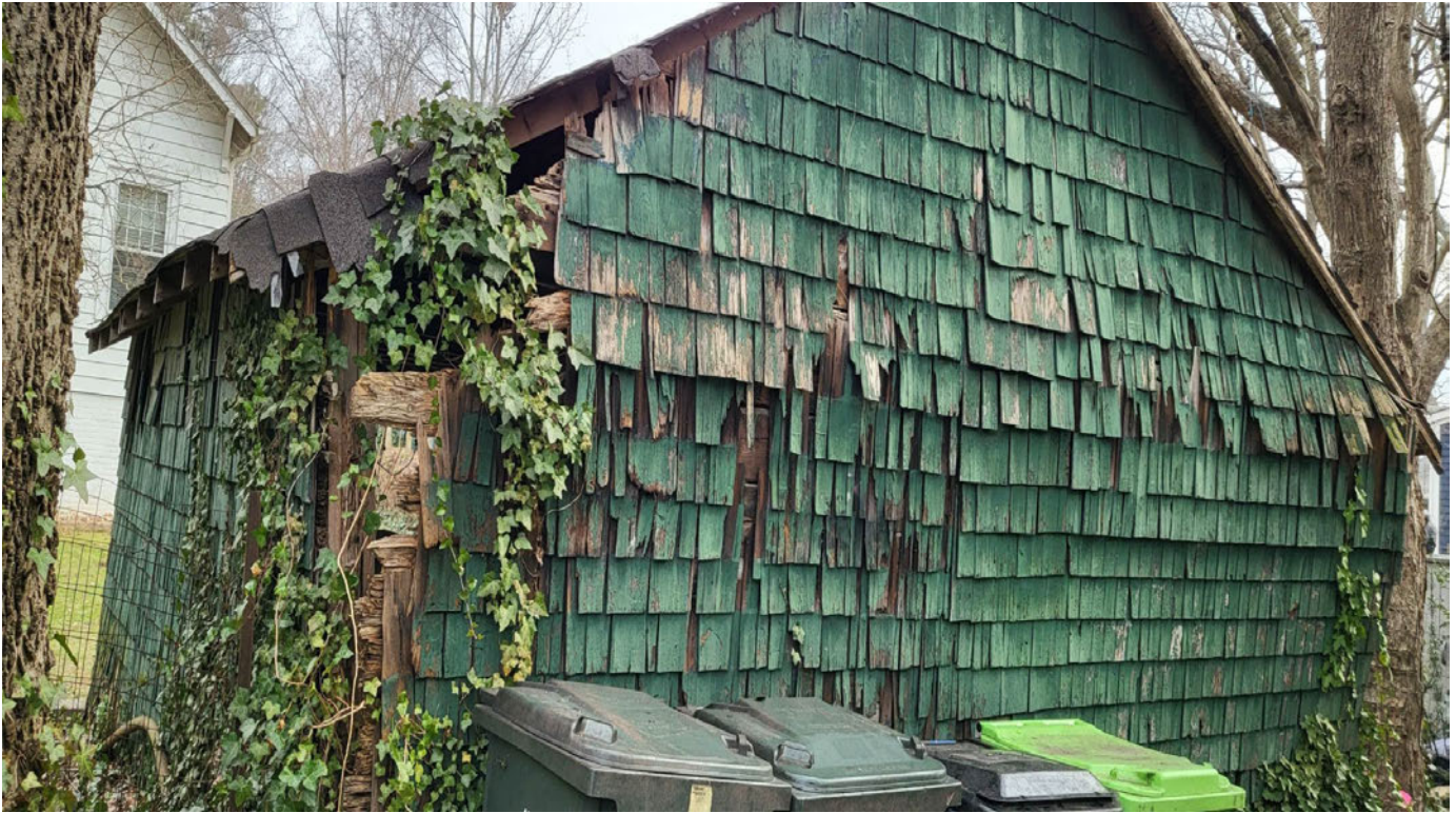
Back view of garage, taken from the alley behind 907 West Lenoir Street
