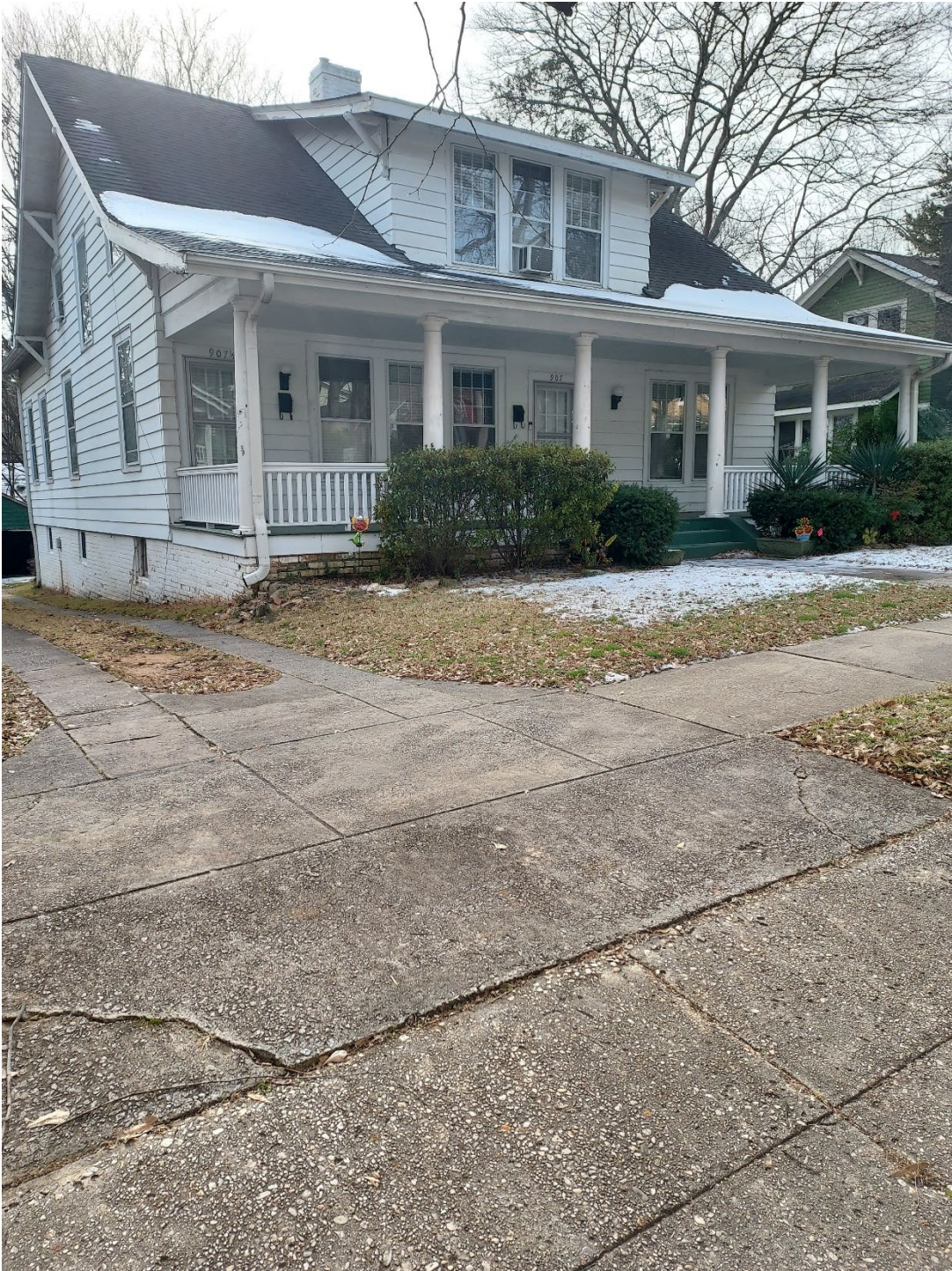
House at 907 West Lenoir Street Raleigh, NC
