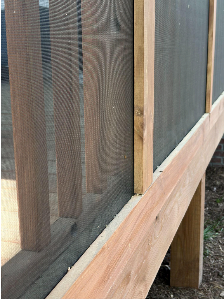
Deck Bug Screen - Detail @ Base
