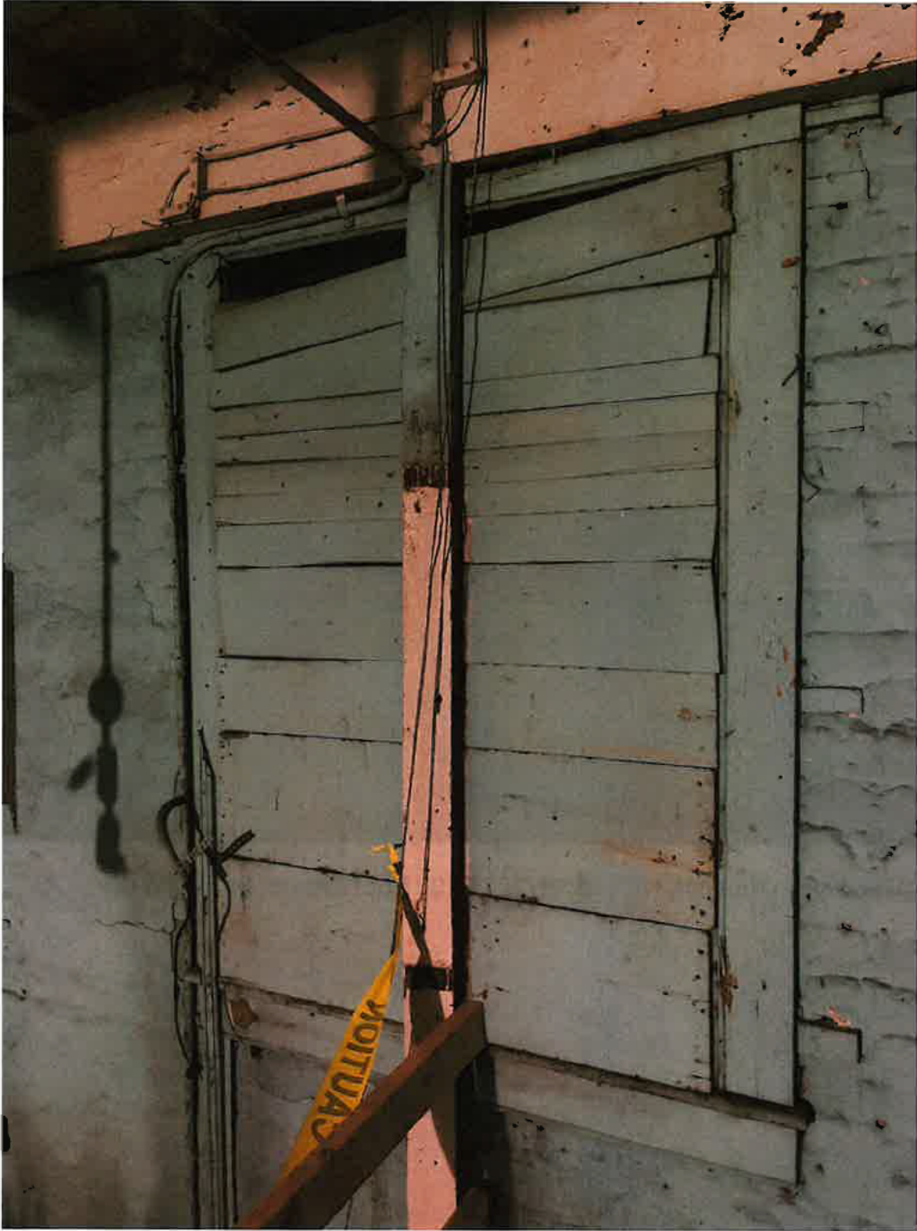
Photo 16: 209 S Wilmington St Raleigh, NC (03/19/2026) 3 rd floor rear bricked in and boarded up window openings with little remaining millwork.
