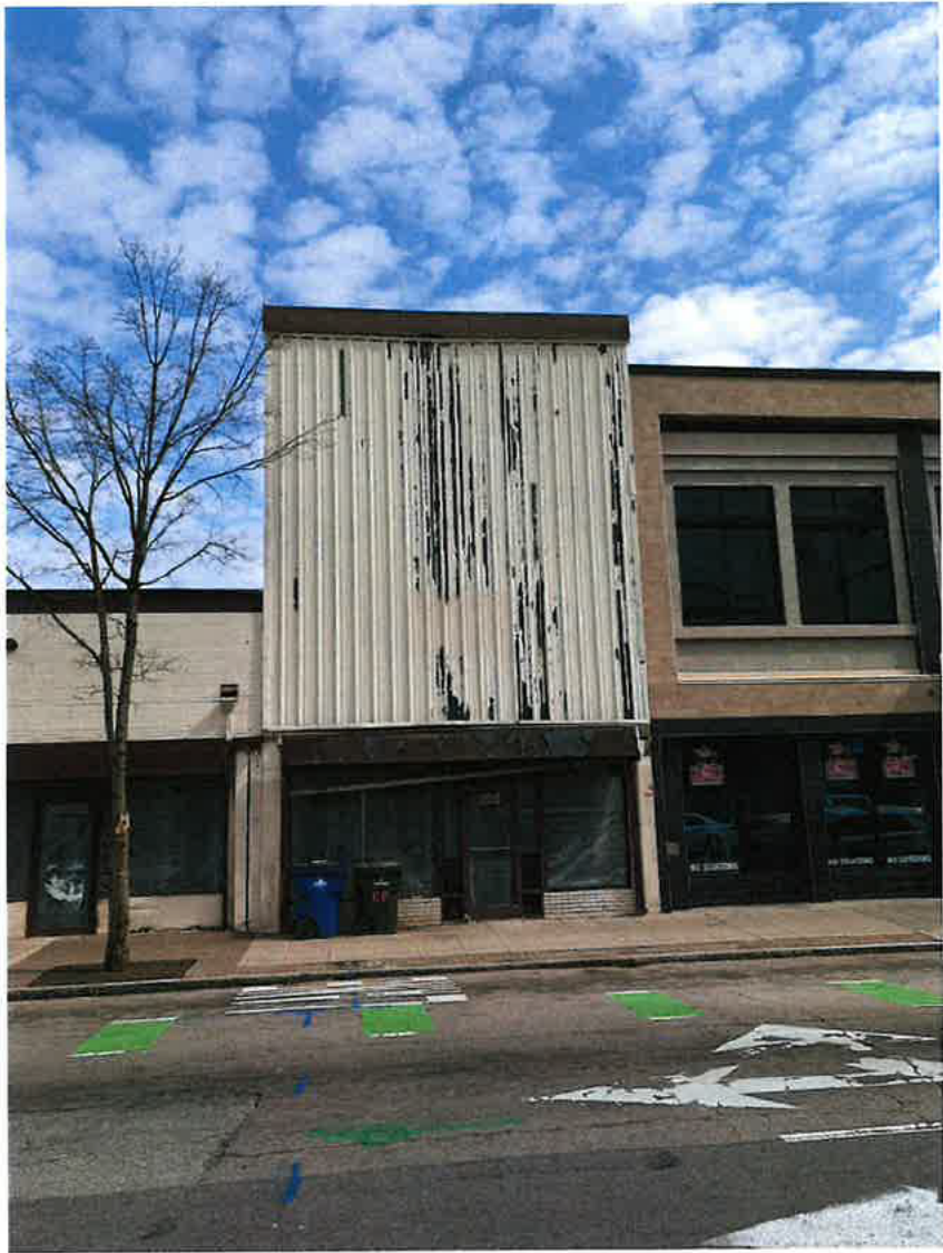
Photo 1: 209 S. Wilmington St Raleigh, NC (03/9/2026) Front Façade
