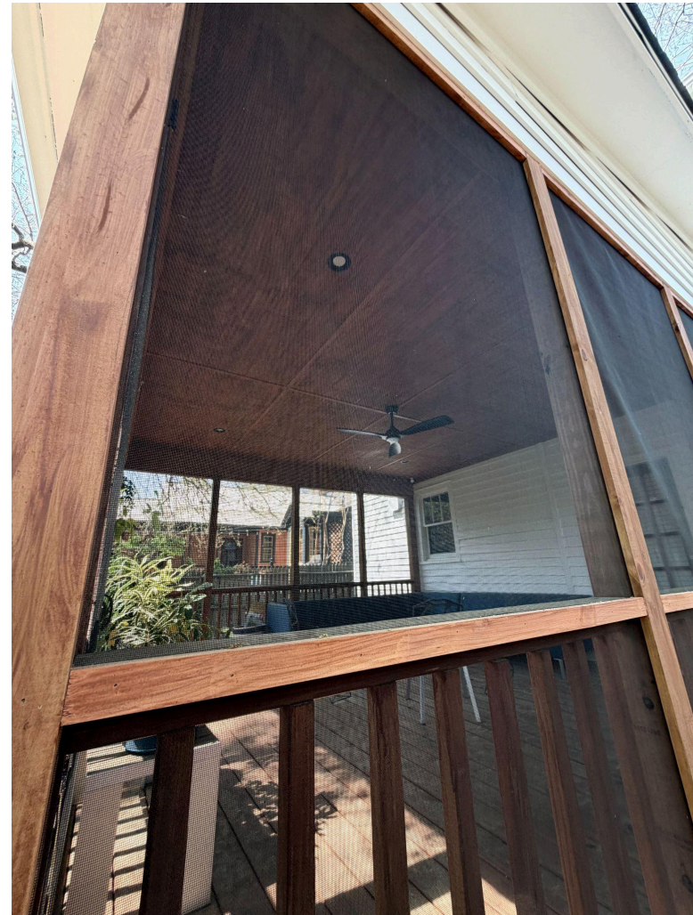
Ceiling Fan + Recessed Cans
