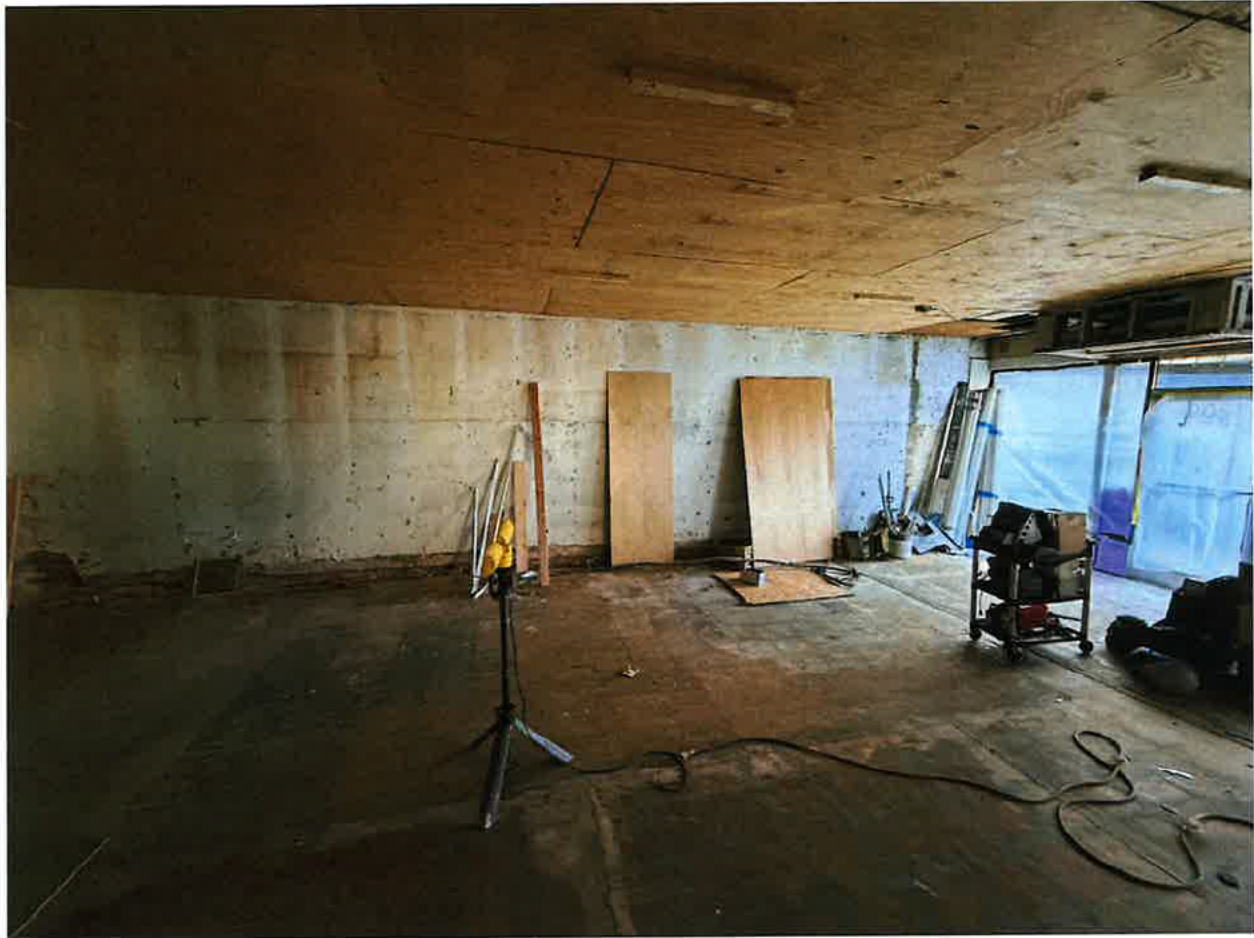
Photo 7: 209 S Wilmington Raleigh, NC (03/19/2026) 1 st floor Interior Facing South West. Appears to be a separate, non-party wall with adjacent 211 S Wilmington St. building.
