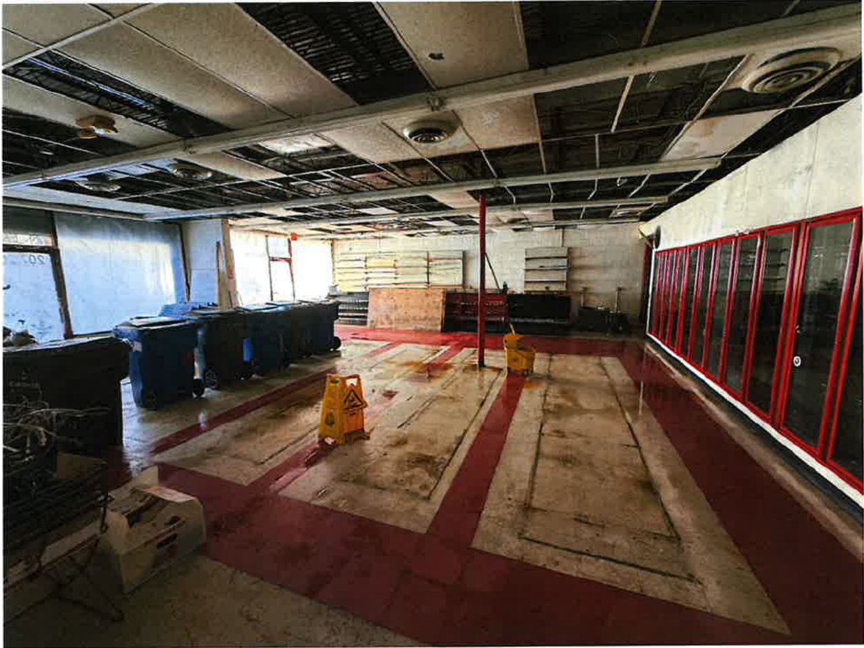
Photo 3: 205 S Wilmington Raleigh, NC (03/19/2026) Interior Facing North toward 201 S. Wimington St.
