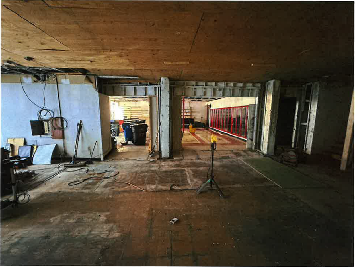
Photo 6: 209 S Wilmington Raleigh, NC (03/19/2026) 1 st floor interior facing North, looking in to 205 . The north masonry wall on the 1 st floor has been removed and replaced with steel columns and beams.
