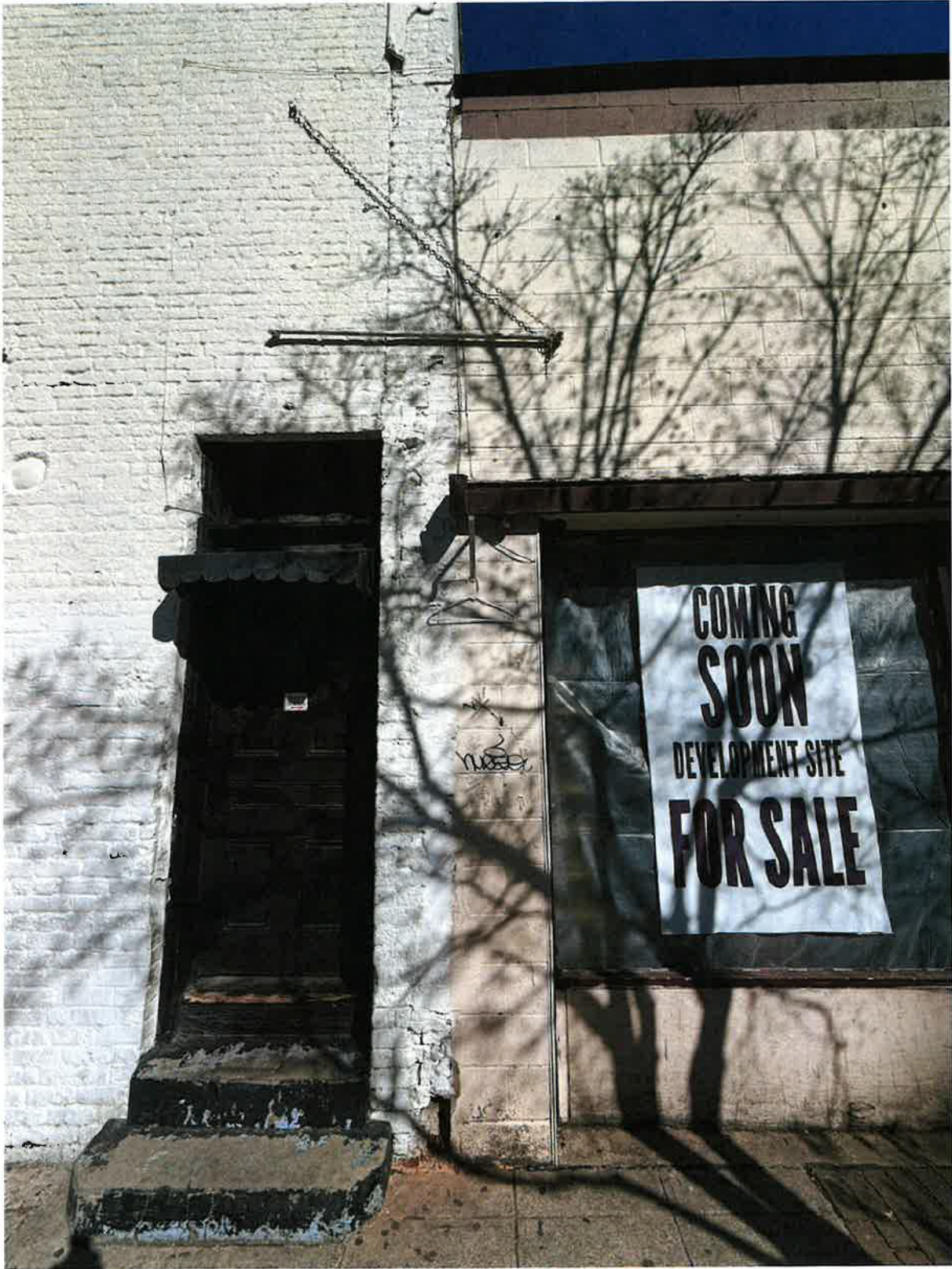
Photo 7: 205 S. Wilmington St Raleigh, NC (03/19/2026) Wall of 201 S. Wilmington independent of 205
