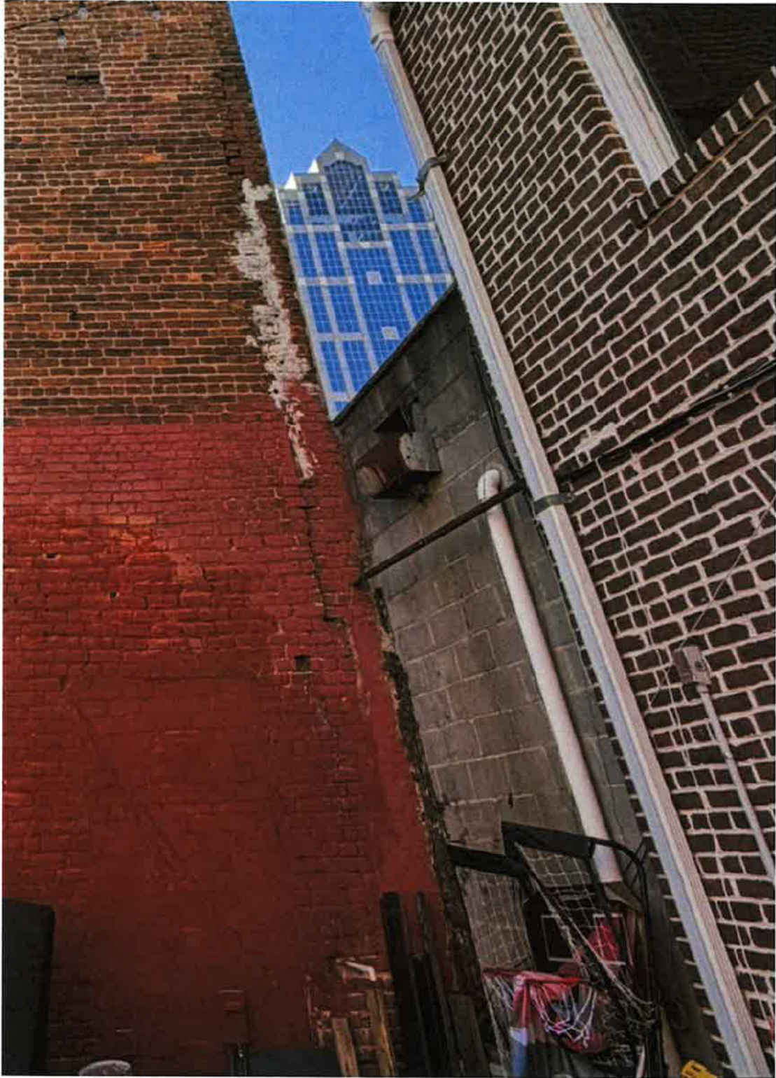
Photo 26: 209 S. Wilmington St Raleigh, NC (03/19/2026) Rear Façade, 209 and 205 separate walls
