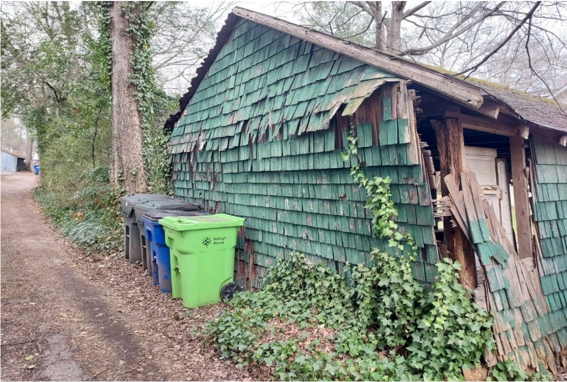
Picture 11 Detached Garage at 907 West Lenoir Street Raleigh, NC
