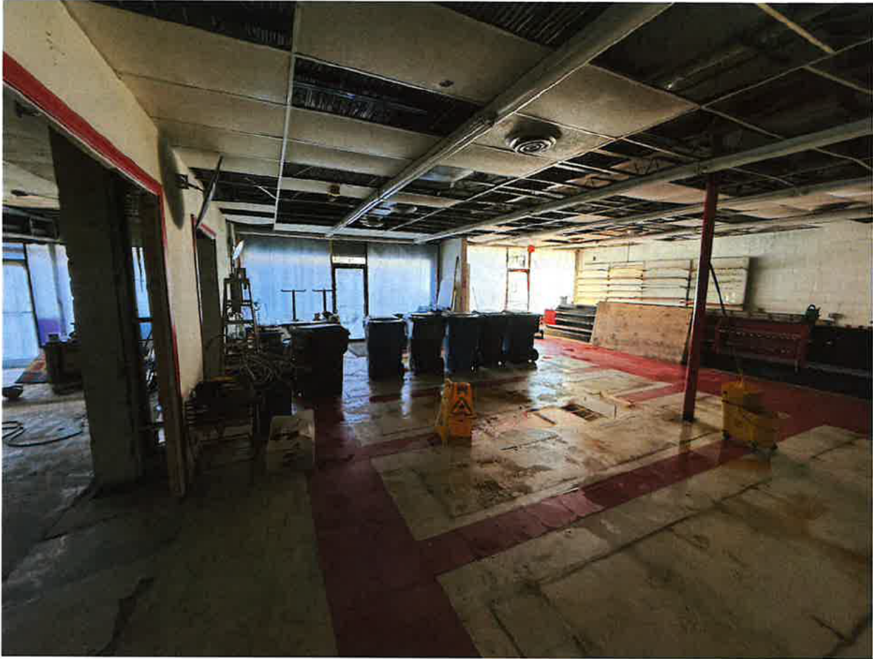
Photo 4: 205 S Wilmington Raleigh, NC (03/19/2026) Interior Facing West toward Wilmington St.
