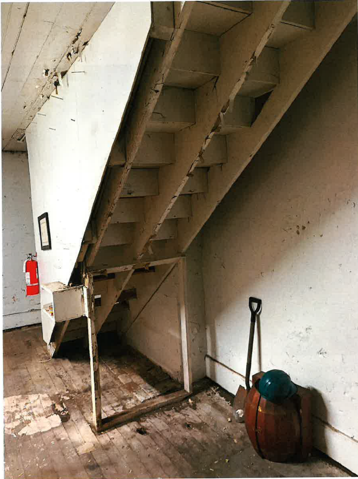
Photo 13: 209 S Wilmington Raleigh, NC (03/19/2026) 2 nd floor, non-original stair to 3 rd floor
