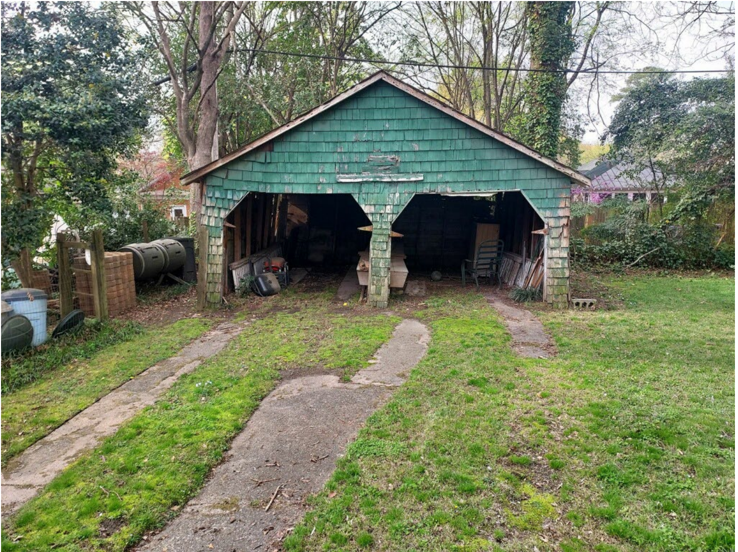
Front view of the detached garage to be demolished
